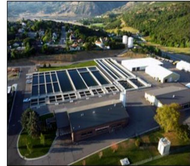
Sedimentation is the second stage of water treatment. The objective of this stage is to remove the floc. This is accomplished as the floc settles out of the water in long sedimentation basins. The cleaner water is
